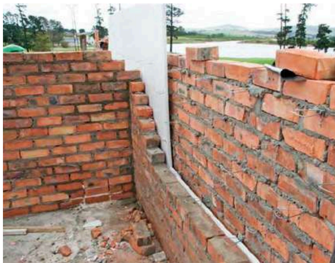
Double layer wall insulation, Maun Hospital
