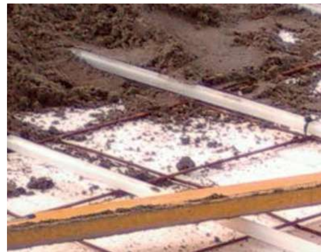
Above slab, below screed insulation
