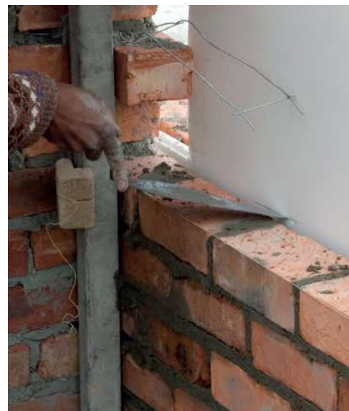
Double layer wall insulation, Maun Hospital
