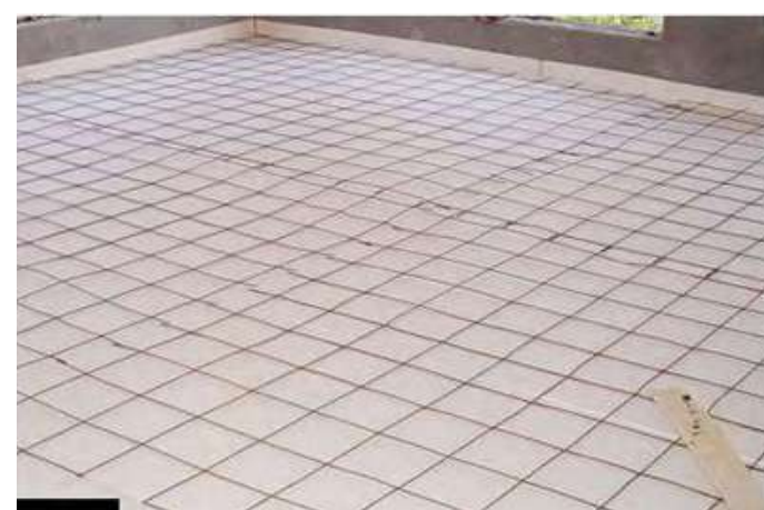
^ IsoBoard installation over slab under screed
