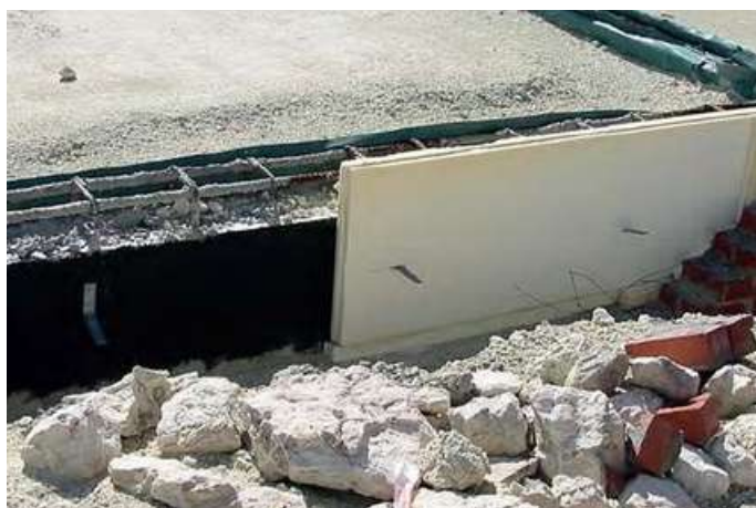
^ Perimeter insulation
