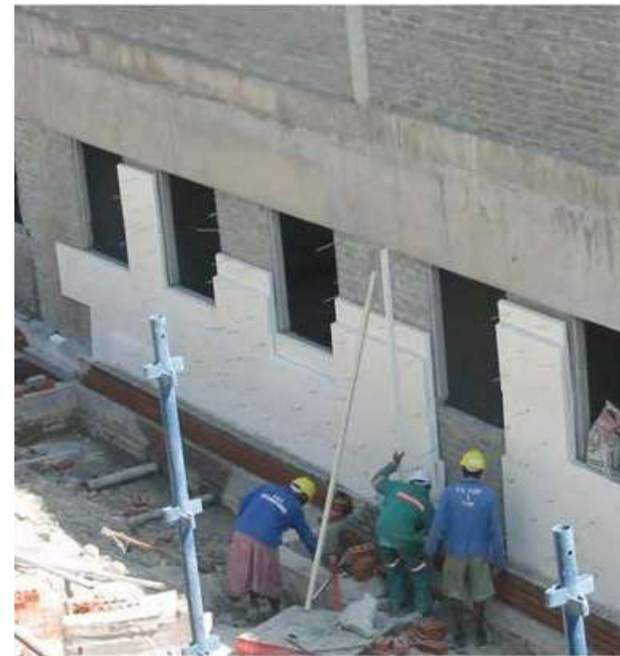
Double layer wall insulation, Maun Hospital
