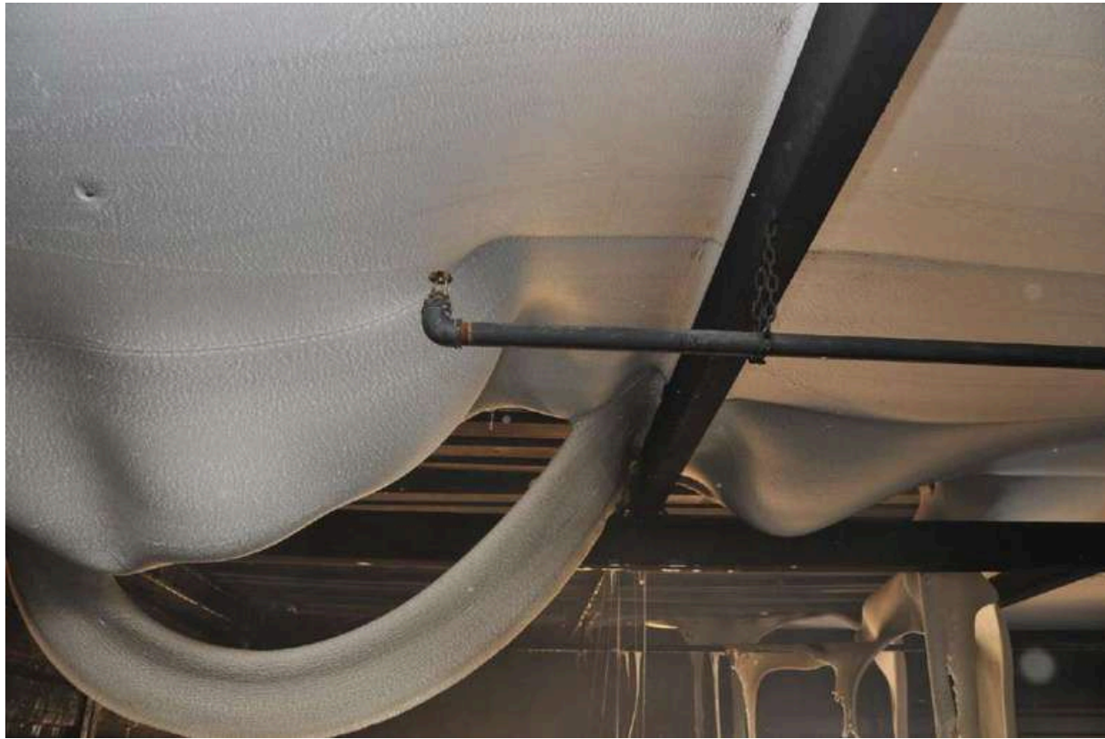
Figure 4.3.9: Material draping close to sprinkler head and over sprinkler pipes in rear
